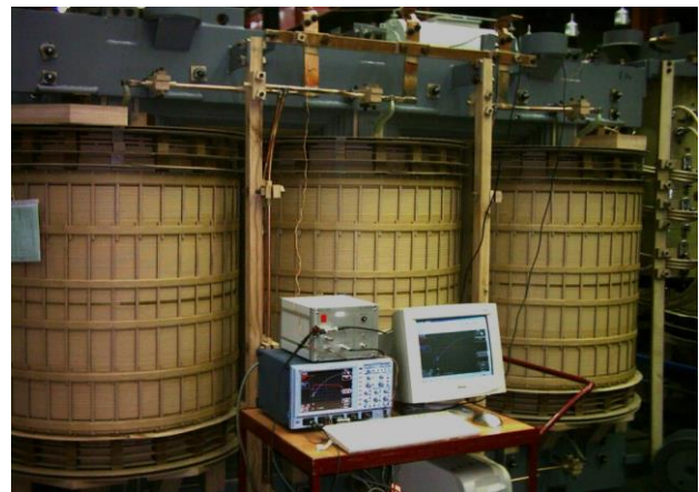
Fig. 1 A view of the transformer active part under test.
