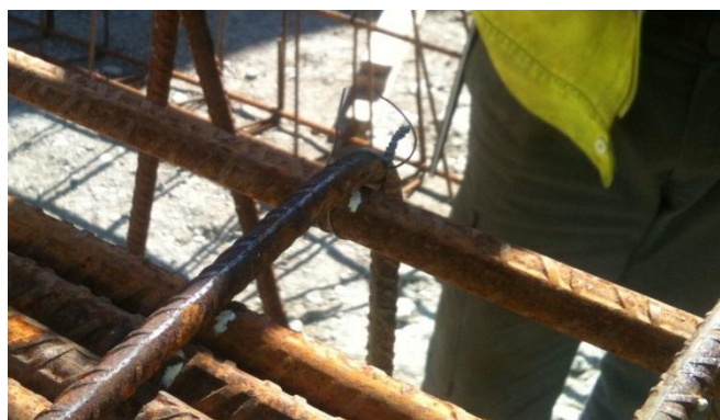
Fig. 5 Close-up of mechanical tying
