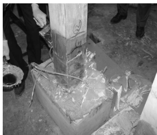
Fig.9 Installation of prefabricated composit sheets
