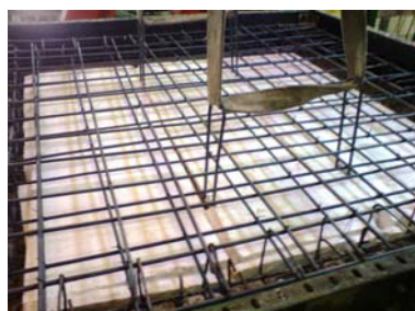
c) Slab reinforcement and hanging support
