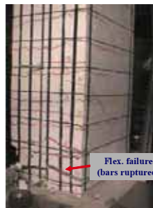
(b) Beam CFB6
