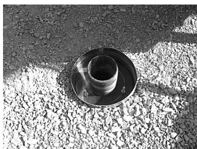
b. backfilling the sleeve with the excavated soil at the considered density
