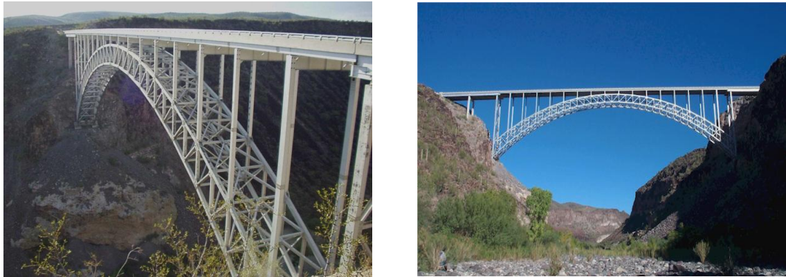
Figure 1. Burro Creek Bridge
