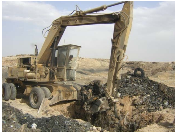
Fig. 2 Excavating the test pit in aged MSW location
