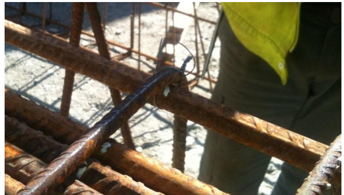
Fig. 5 Close-up of mechanical tying
