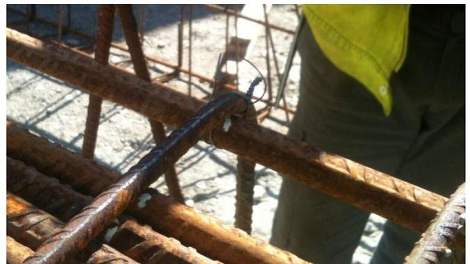
Fig. 5 Close-up of mechanical tying
