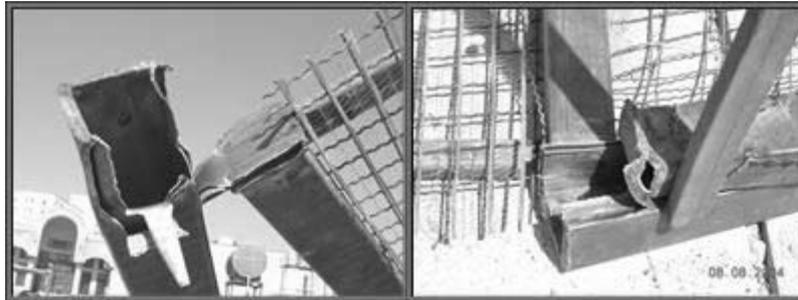
**Fig.7** Destruction of beam to column moment connection
