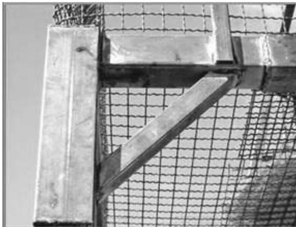
**Fig.10** Using corbels for strengthening the connections
